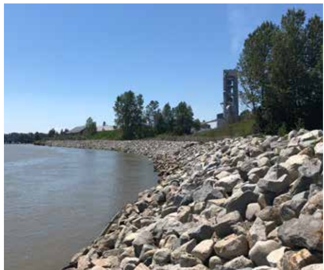
Flood management work
