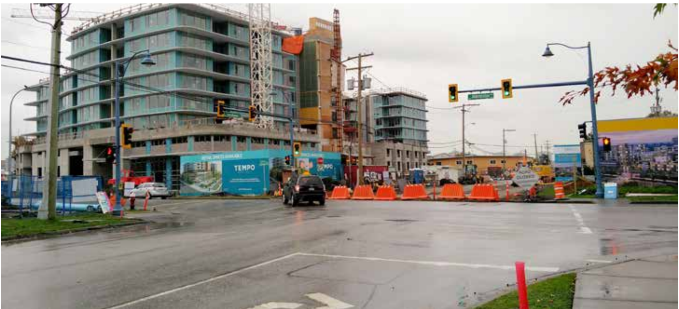
Servicing Agreements and Development Cost Charges address infrastructure needs and provide amenities for a growing population.
