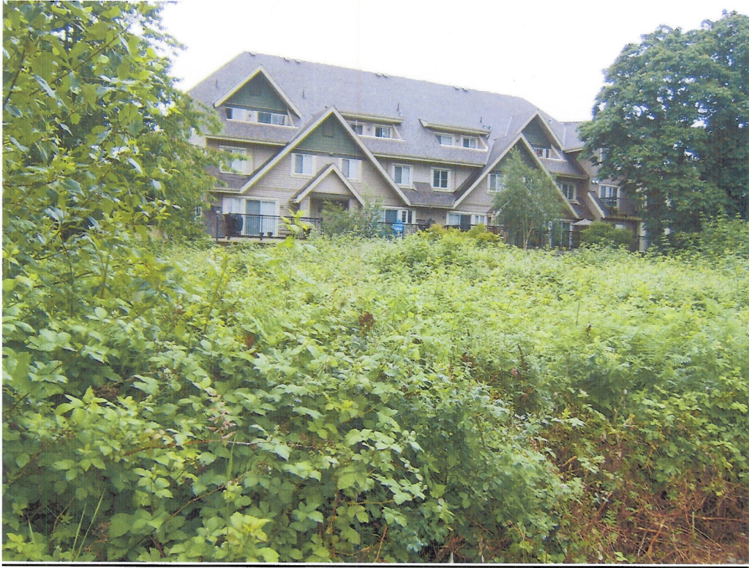
Address: 9271 Alberta Road- Rear Yard view Taken by Ron Graham June 10 th , 2010.
