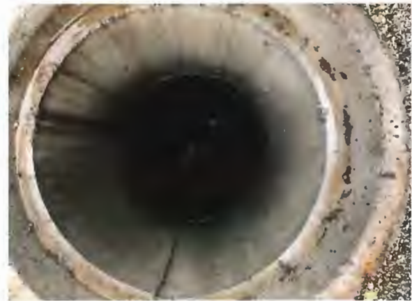
January 24, 2020 – 90-degree vertical bend service connection
