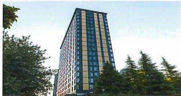
Figure 3: Brock Commons, UBC, in Vancouver, BC
