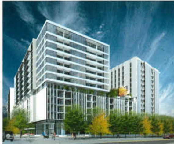
Figure 2: Moderate ratio of window to wall area represented.
