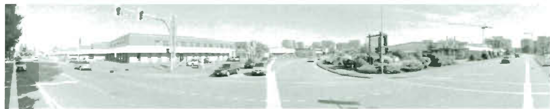
5 Alderbridge Way and Minoru Blvd Intersection
