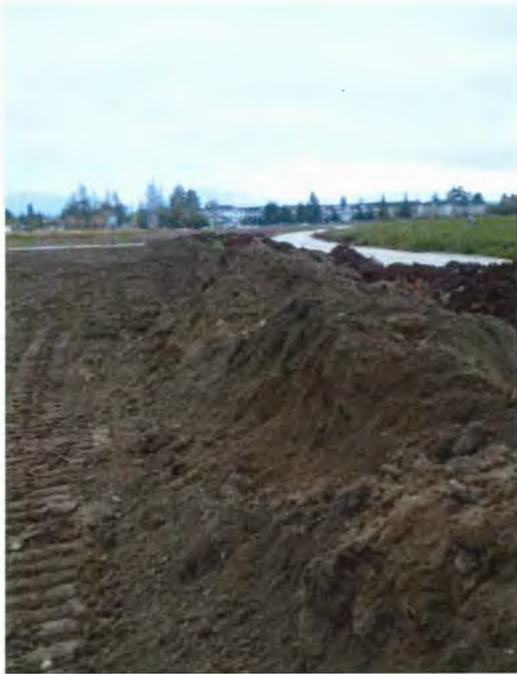
Figure 5 Topsoil stockpile July 27, 2017
