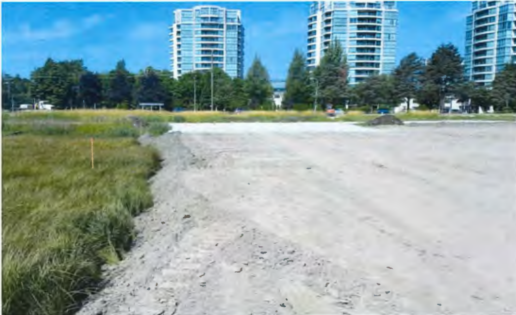
Phase 1 Fill deposition completion, southwest corner
