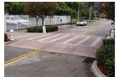
INSPIRATION: Primary pedestrian routes should be continuous through vehicle circulation areas, considering marked and raised crosswalks where these uses intersect.
