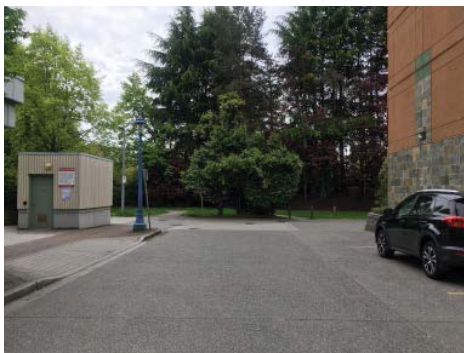
TODAY: The existing Alderbridge Gate entry from Westminster Highway provides little invitation into Minoru Park.
