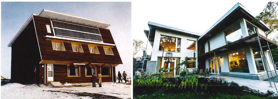
Figure 2 – LEFT: Saskatchewan Conservation House (Regina, SK, 1977) [Source: passipedia.org] RIGHT: Bernhardt Passive House (Victoria, BC, 2013) [Source: Passive House Canada (courtesy of D. Ford)]
