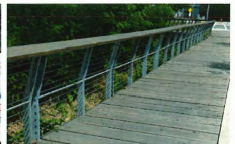
Existing railing at River Road boardwalk
