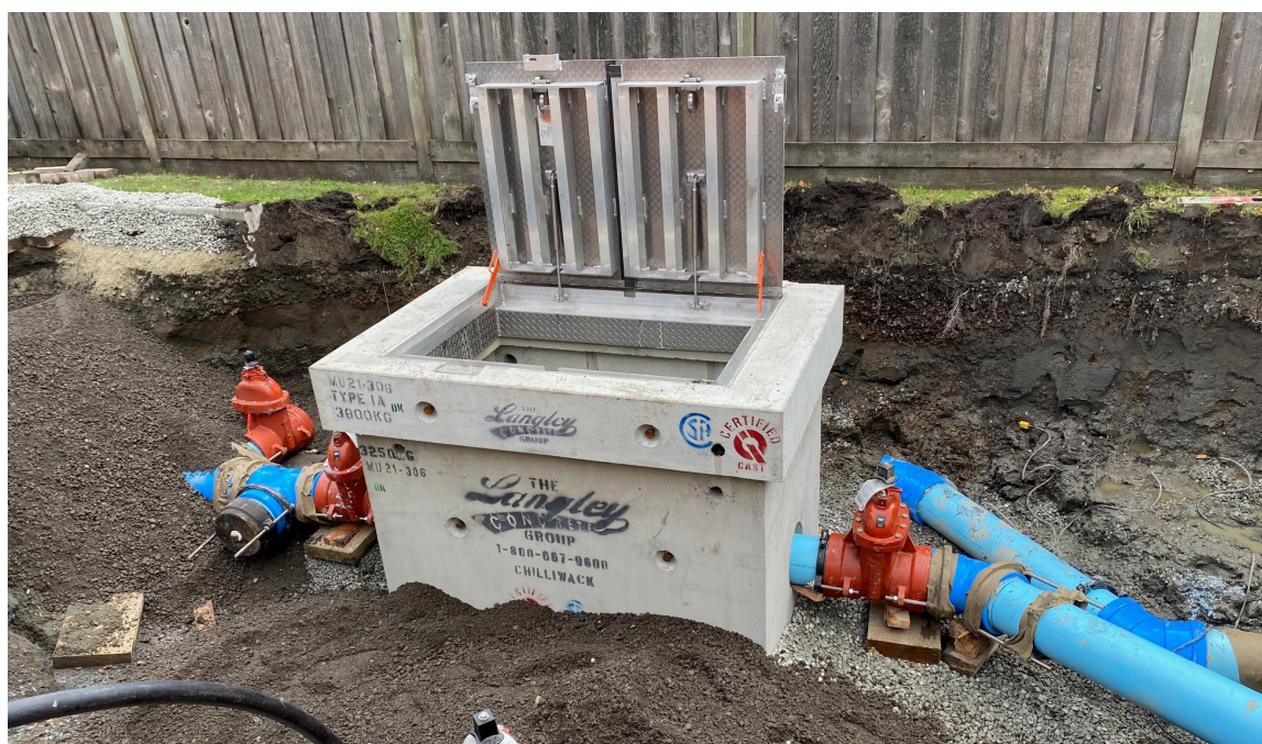
Multi-Family Water Meter Installation
