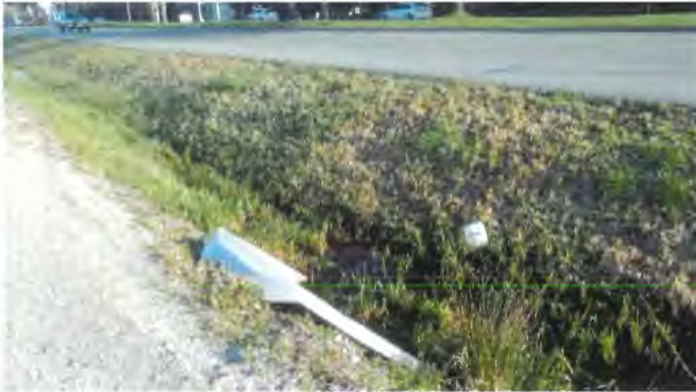
Figure 3-5: South Ditch looking upstream from outlet headwall.
