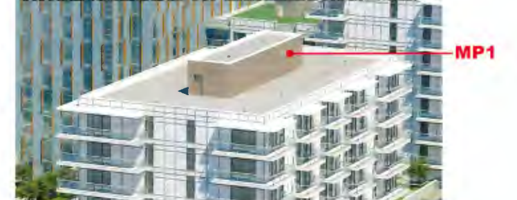
TYPICAL TOWER ROOF TOP WITH ELEVATOR OVERRUN
