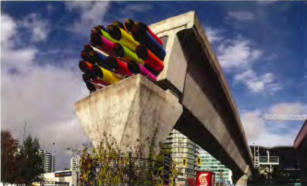
Figure 4. Cluster , Carlyn Yandle, 2014. Richmond-Brighouse Canada Line Terminus Station.
