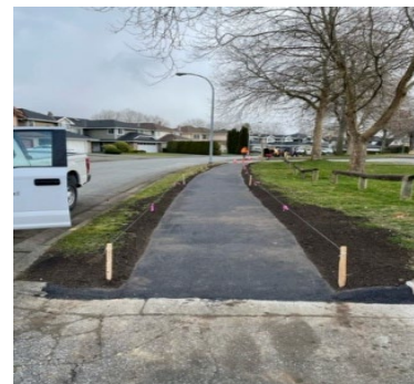
Figure 1: Talmey School Walkway
