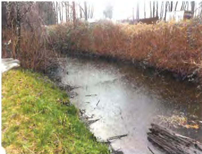
PHOTO 11: DITCH LOCATED AT 17260 RIVER ROAD - NOTE WATER LEVELS ARE QUITE HIGH. THIS PHOTO WAS TAKEN JANUARY 7, 2020
