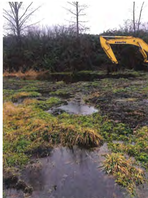
PHOTO 5: FACING DUE WEST ON THE PROPERTY. THIS STANDING WATER IS OVER 0.3 M DEEP.
