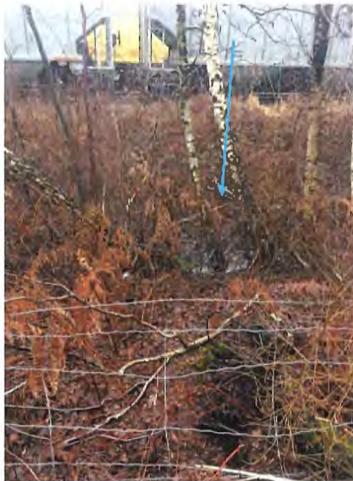
PHOTO 10: DITCH SITUATED BETWEEN THE CN RAILWAY AND THE PROPERTY, WHICH IS THE FENCE IN THE FOREGROUND. THE WATER LEVELS ARE INDICATED BY A BLUE ARROW.
