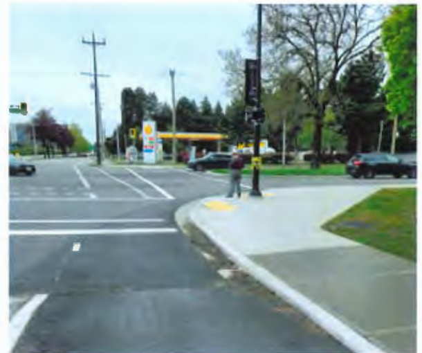
Figure 2: Southbound Garden City Rd @ Lansdowne Rd Before: Channelized Right-Turn Island / After: Standard Intersection with Separated Cycling Facilities
