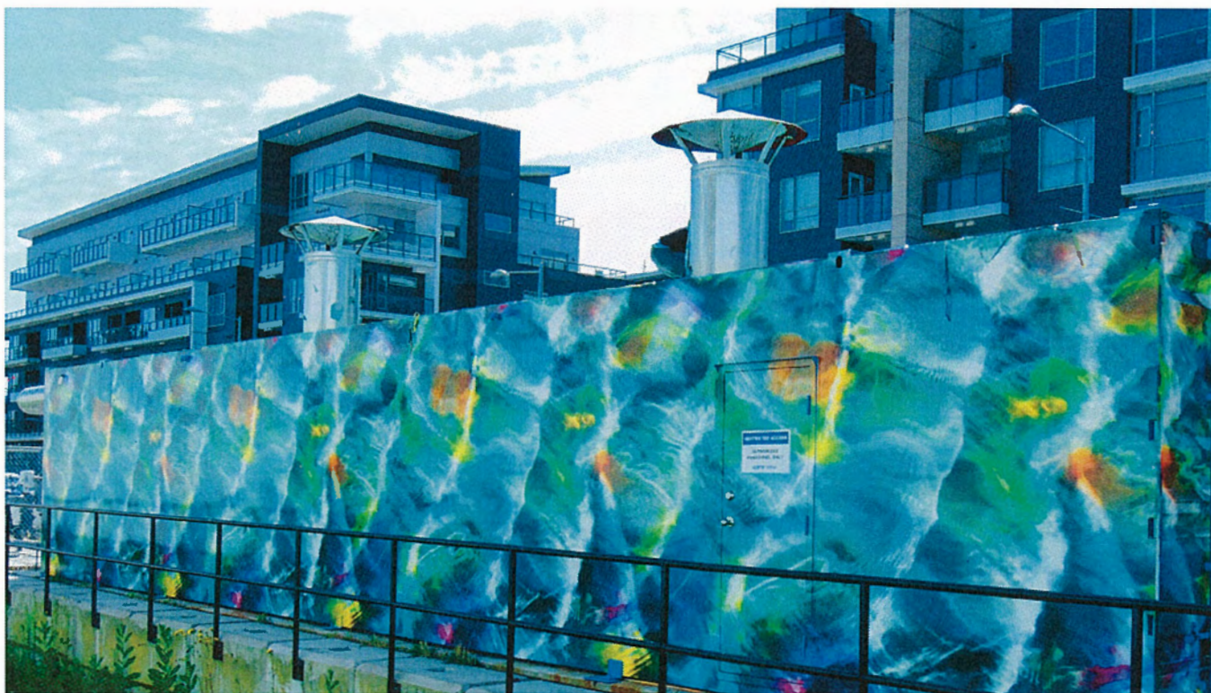
Oval Village District Energy Utility Interim Energy Centre Public art feature: Underwater (2017) by Andrea Sirois
