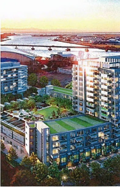
The River Park Place 2 development will be connected to the Oval Village District Energy Utility in 2019, providing 298 residential units with domestic hot water and heating services
