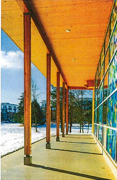
Covered deck for public use at the Alexandra District Energy Utility Energy Centre
