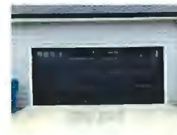
12. METAL GARAGE DOOR & MAN-DOOR BM - HEARTHSTONE CC-1601
