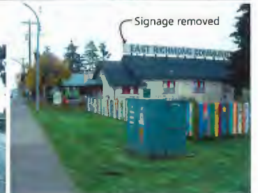
Lack clear of signage and information
