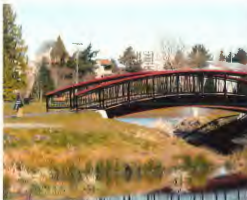
Bridge over The Hollow
