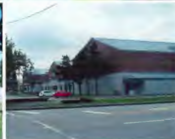
Major intersection - no signage and 'back' end of building
