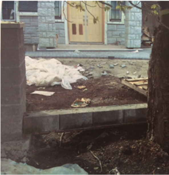
Construction of a Floating Grade Beam
