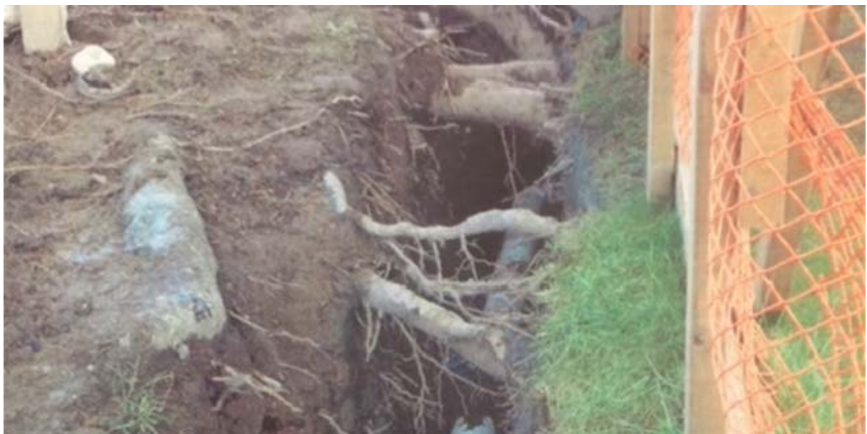
Hydro Vac to install services without cutting roots
