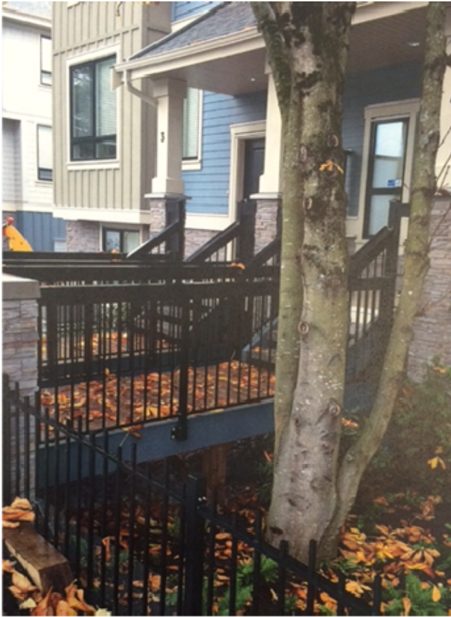
Bridging grade changes to retain existing trees
