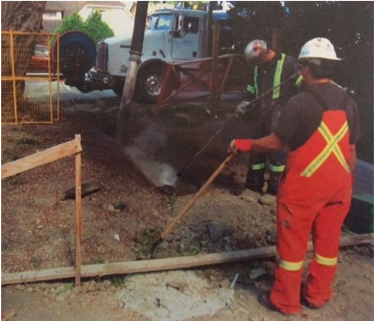
Hydro Vac (High pressure water excavation)
