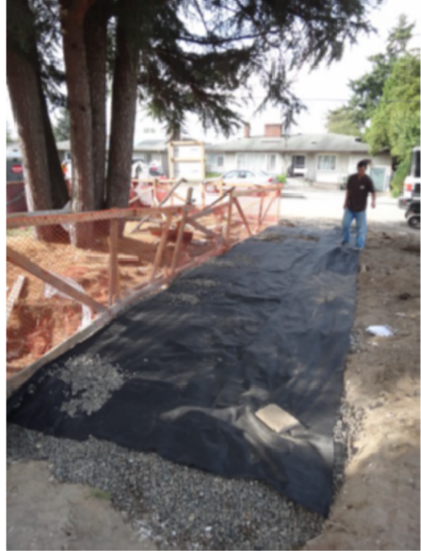
Gravel and landscape fabric over perforated tubes
