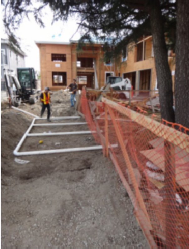
Aeration tube layout for driveway encroachment
