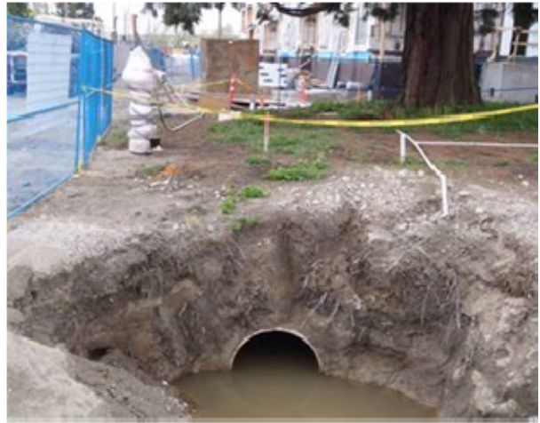
Pipe installed for services under tree root zone
