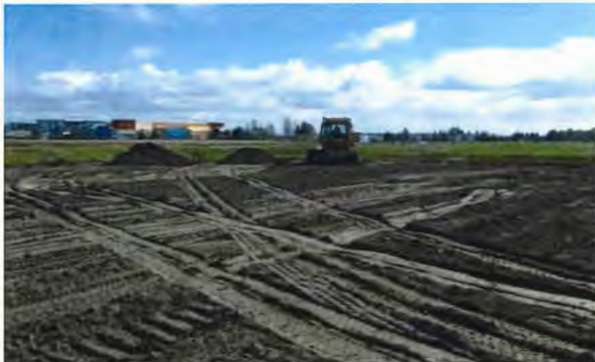
Figure 4 Soil being graded with dozer June 28, 2017
