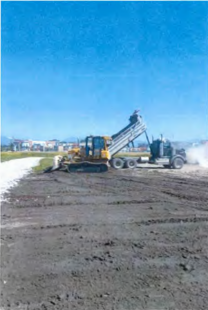
Figure 6 Fill being deposited July 6, 2017
