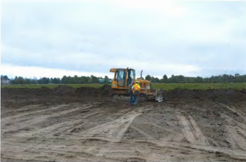
Figure 4 Soil being deposited July 27,2017
