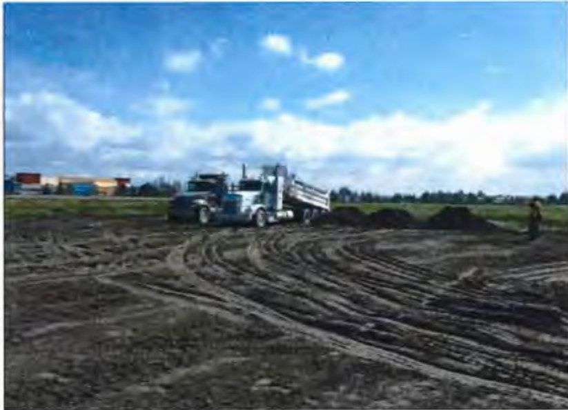
Figure 3 Soil being deposited June 28, 2017
