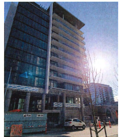
A development in the Oval Village nearly ready to connect to the DEU.
