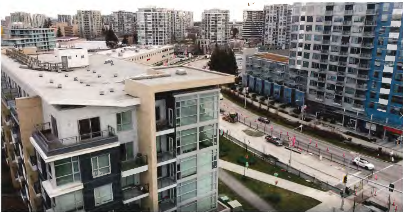
Distribution piping being implemented to connect another building to the OVDEU.
