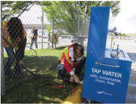
Water Services crew setting up the Tap Water Station
