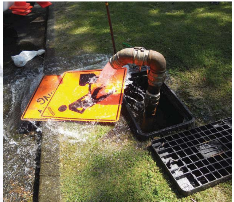
Water Services staff flushing the main line as part of the low flow flushing program
