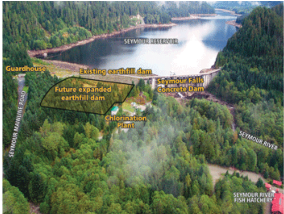
Seymour Capilano Water Filtration Projects
