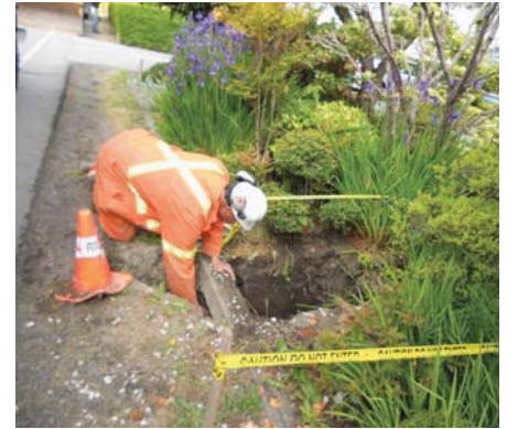
Water Meter Installation
