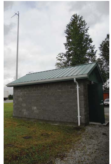
Pressure-reducing valve station that connects to S.C.A.D.A. telemetry system
