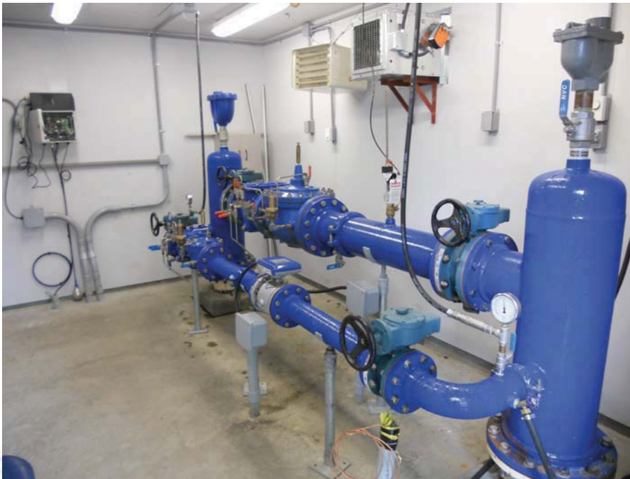
Inside the pressure-reducing valve station
