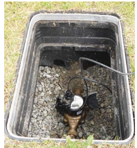
Installed water meter
