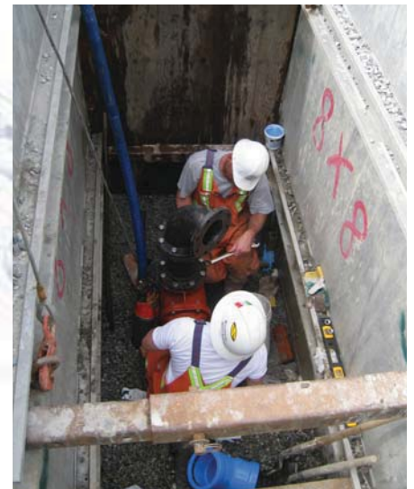
Water Services crew upgrading an existing supply line
