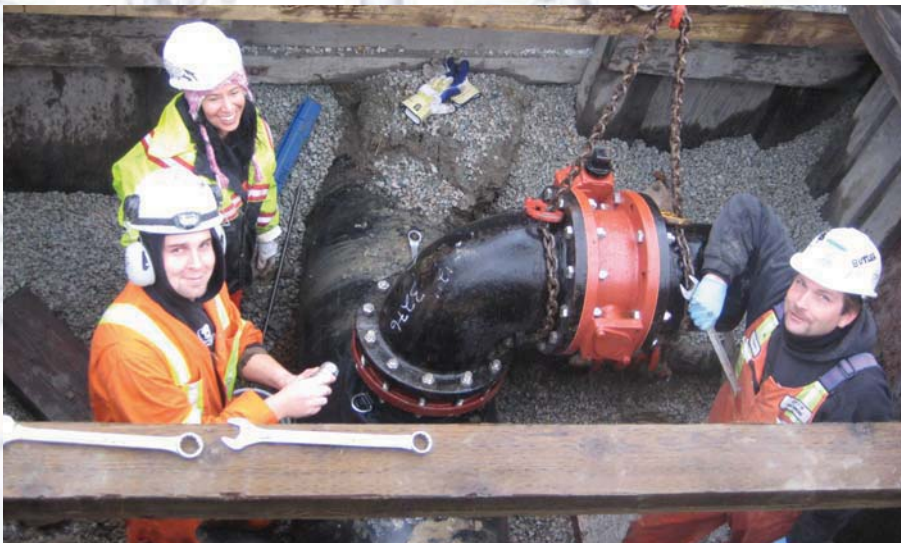
Water Services crew installing a large residential/commercial water supply line.
