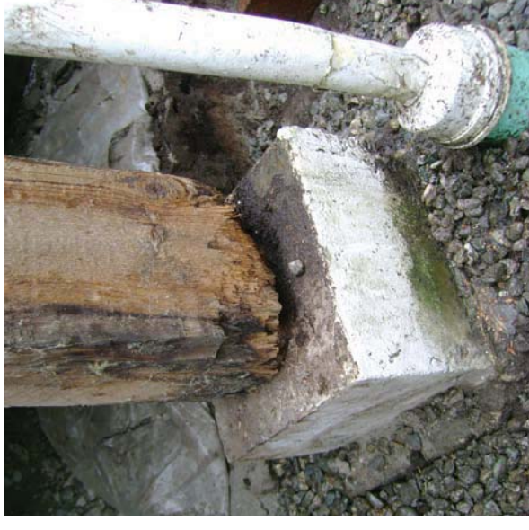
London Farmhouse Foundation
