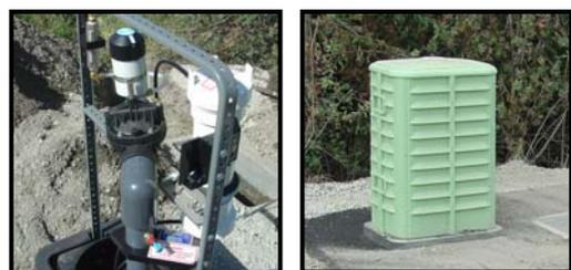
Automatic Flushing Station and cover
