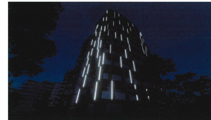
Night View of Light Feature
