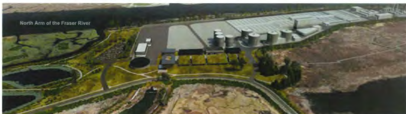
Rendering showing view of the new IWWTP from the south; the planted slope of Area 18 (perimeter screening strategy "E") of Area 18 is along the east half of the plant. Not visible in this rendering is the steel screen fence (perimeter screening strategy "B") for this area, and the short retaining wall to help make up the grade change.
