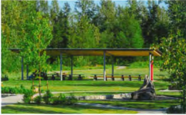
Picnic shelter precedent at Surrey Bend Regional Park (Photo: Matthew Woodruff, Local Practice, photo used with permission)
