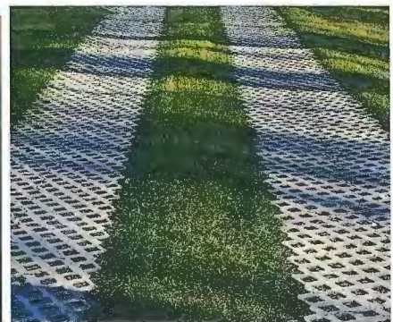
Concrete Pavers Option (Structural grass)
