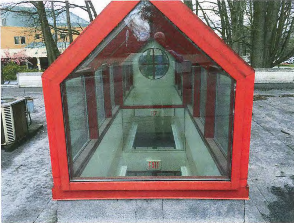
Picture 4 - Aluminum Framed Skylights
