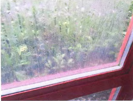
Figure 33 – Failed IGU.
