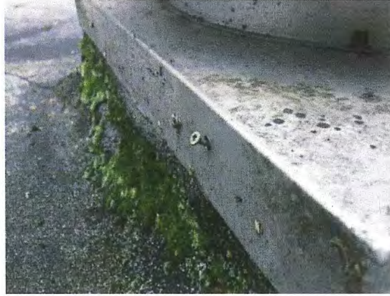
Figure 78 – Unsealed fasteners at extraction fan.
