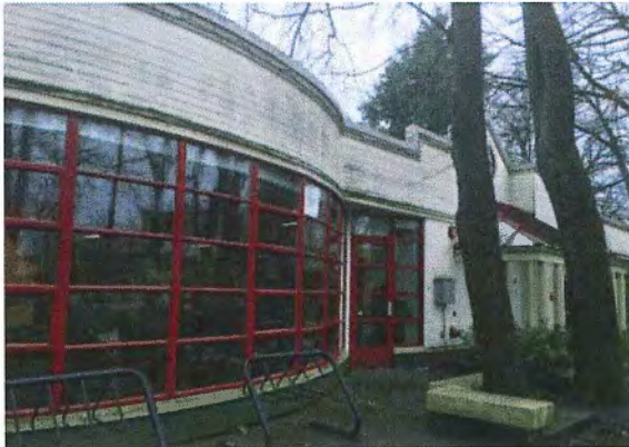
Figure 3 – Partial View of North-east Elevation.
