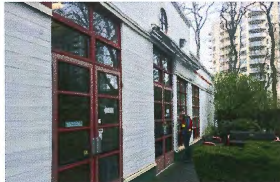
Figure 43 – Exposed doors at the storefront system.
