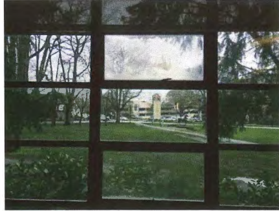
Figure 34 – Failed IGUs
