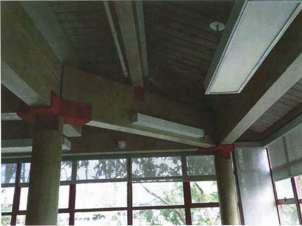
Picture 1 - Exposed Timber Roof Framing
