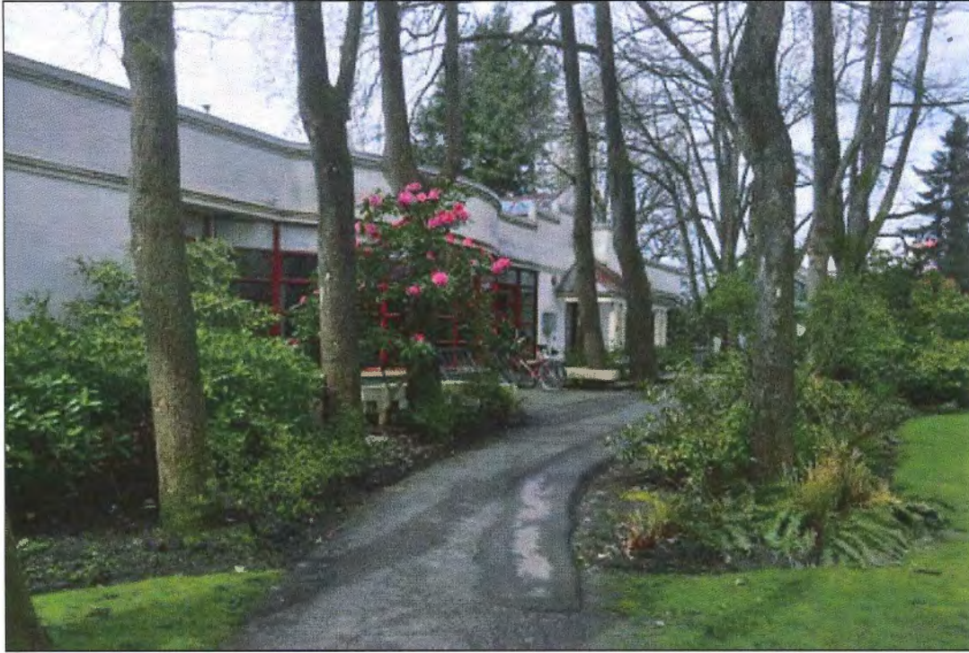
Figure 2: Proximity of individual tree specimens to the entrance and circulation routes leading to the Seniors Centre.
