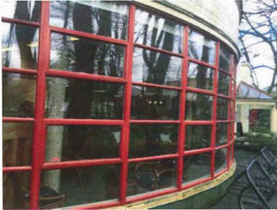
Figure 29 – Aluminum-framed windows with rolled-in glazing stops.
