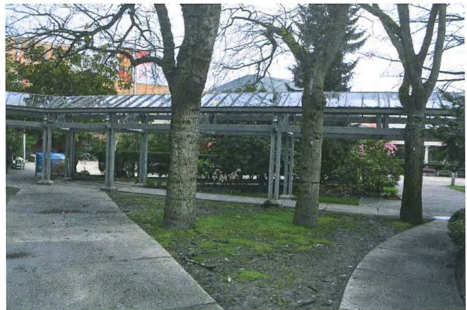
View from west side of MPAC showing visibility obscured by bushes and covered walkway.
