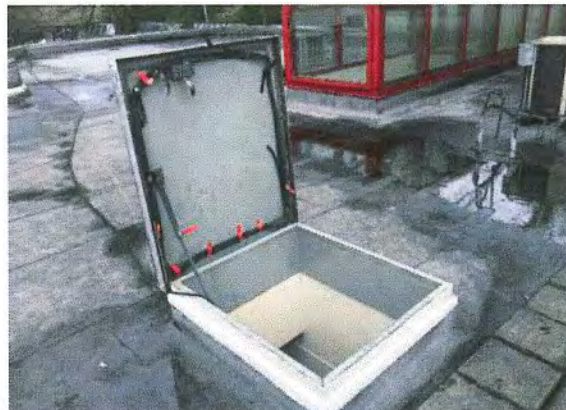
Figure 80 – Roof access hatch.
