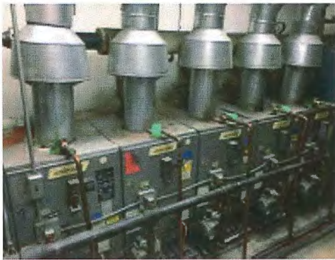
Figure 1 – Existing Boilers
