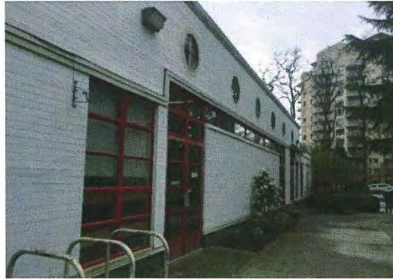
Figure 4 – Partial View of West Elevation.
