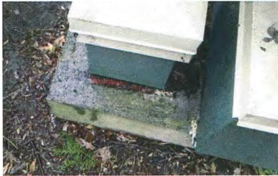
Figure 15 – Typical base of exterior column.
