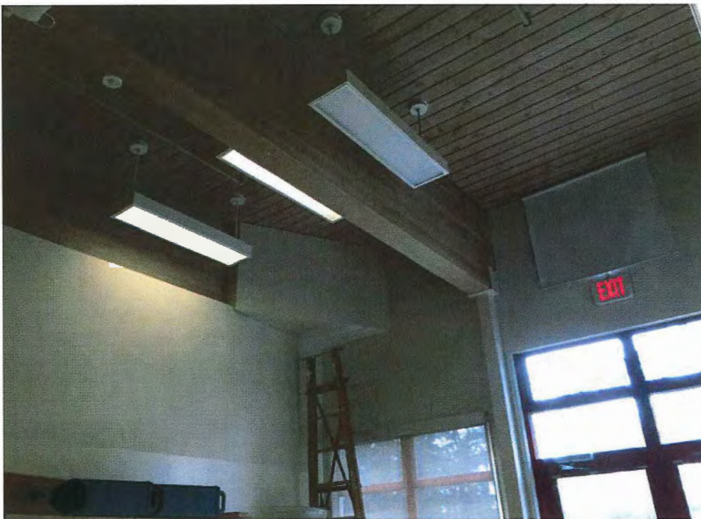
Picture 2 - Glulam Beams Clearspan Activity Room
