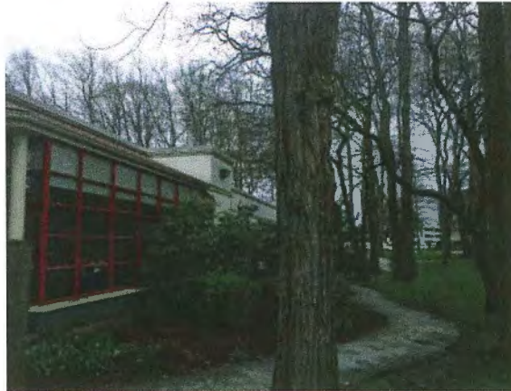
Figure 7– Partial View of South-east Elevation.
