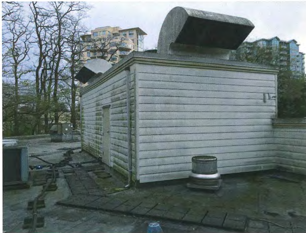
Picture 3 - Mechanical Penthouse with adjacent roof step over Activity Room
