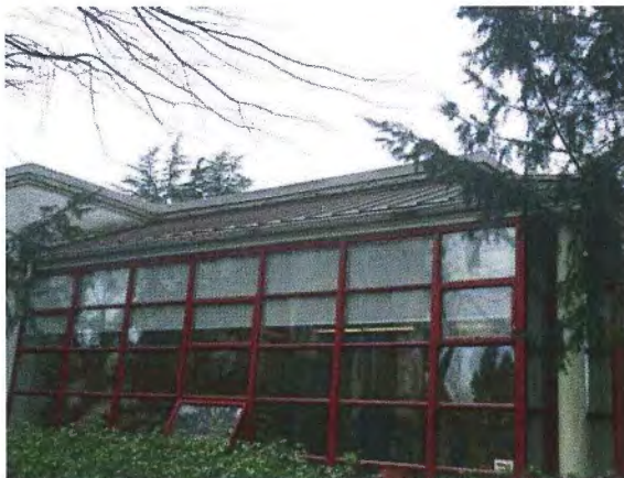
Figure 61 – Standing seam metal sloped roof.
