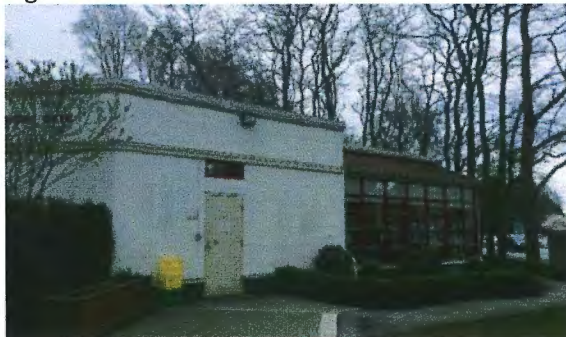
Figure 5 – Partial View of South-west Elevation.
