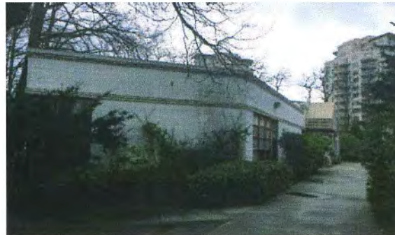
Figure 6 – Partial View of North-west Elevation.
