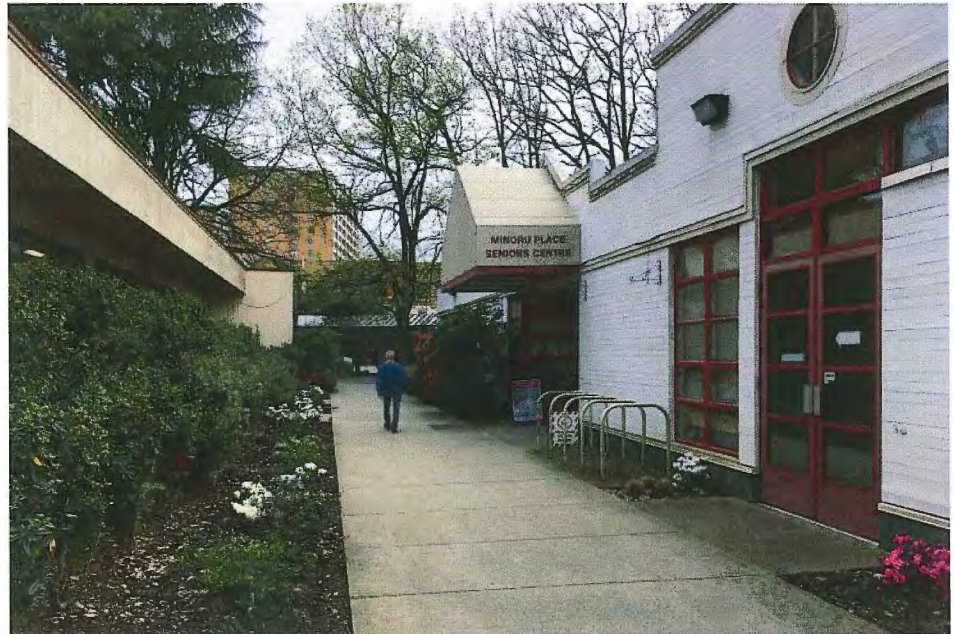
View of west walkway indicating need to update and highlight the building entry.
