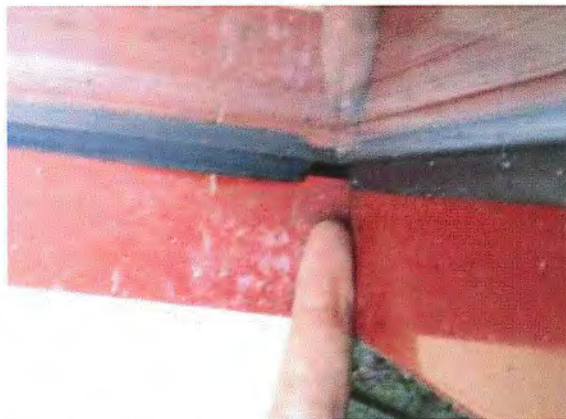
Figure 36 – Shrunken gasket at a window.
