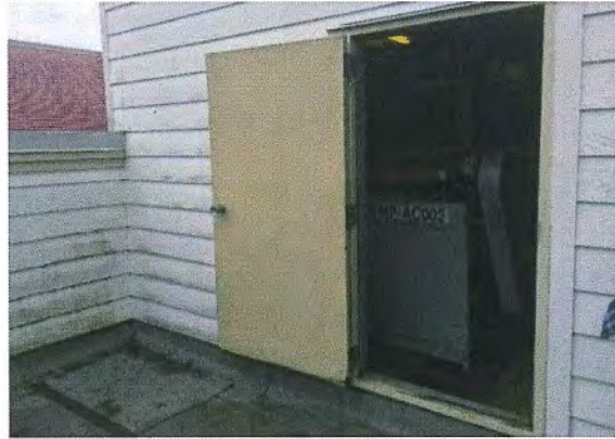
Figure 40 – Wood door slab at the mechanical room.
