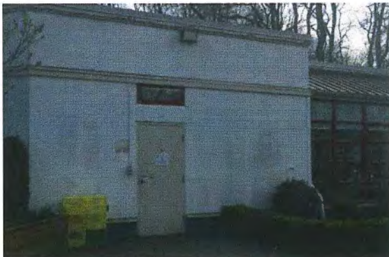
Figure 42 – Exposed pressed steel door.
