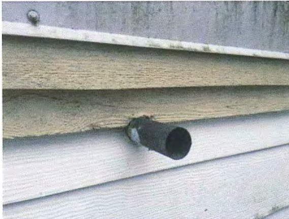
Figure 54 – Wall penetration (typical).
