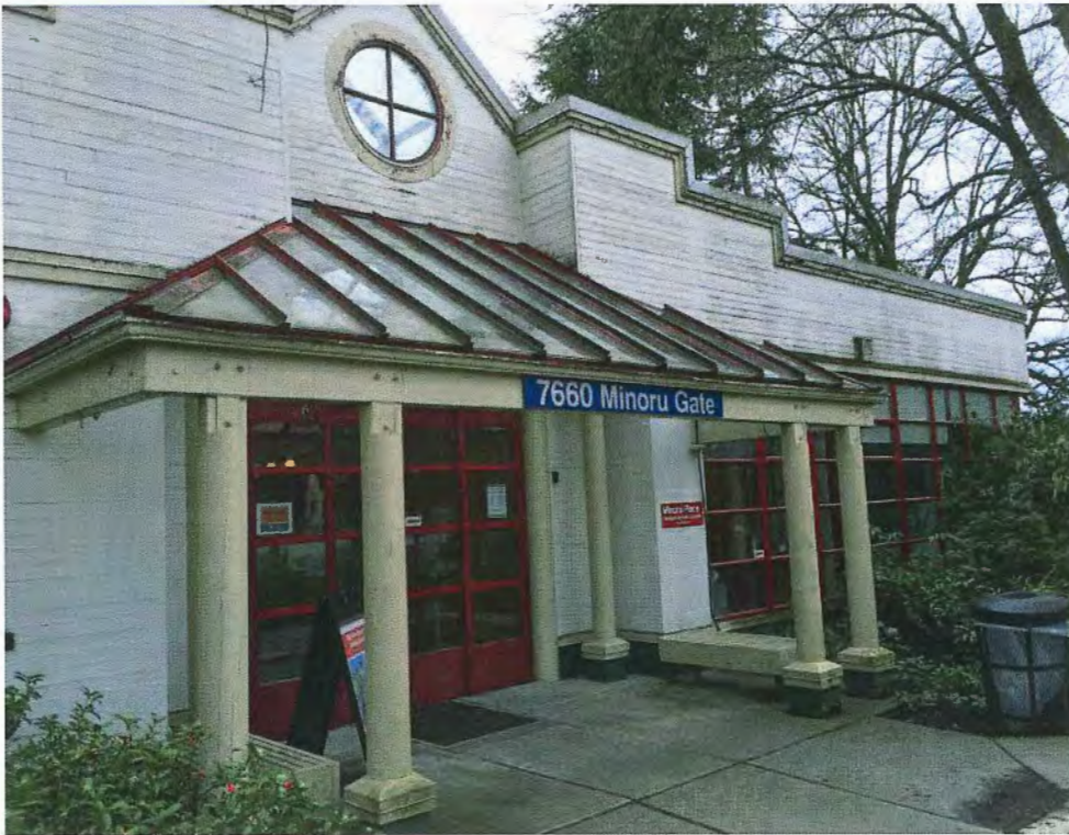
Picture 5 - Building Exterior in Fair Condition – requires cleaning and painting
