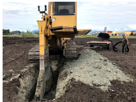
Drain tile installation, June 2018
