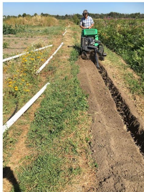
Irrigation line installation, July 2020
