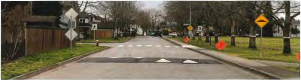
Figure 1: Installation of Speed Humps on Fundy Drive
