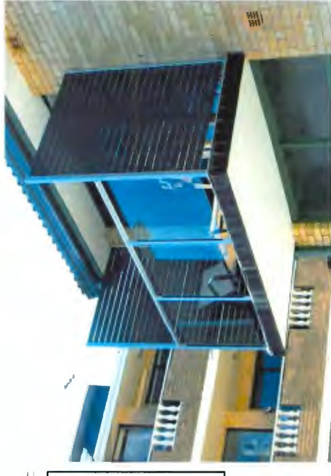
PRIVACY SCREEN SAMPLE -ALUMINUM POSTS -COMPOSITE HORIZONTAL SLATS -TO BE FACE MOUNTED TO PONY WALL
