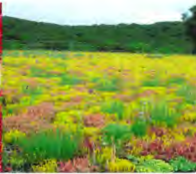
L8/L11 Sedum green roof
