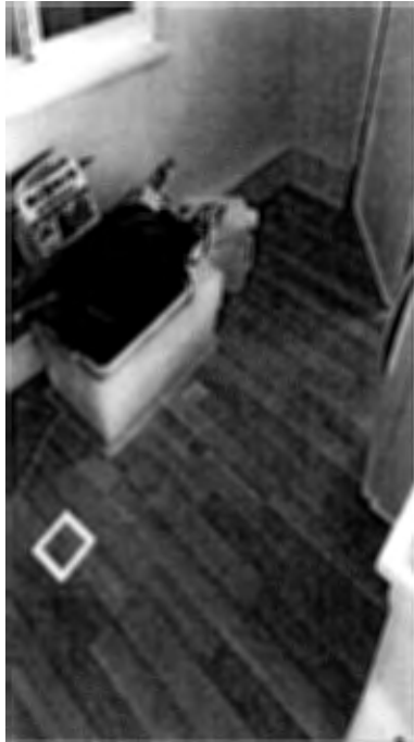
Photo 9: Laundry Room Floor
