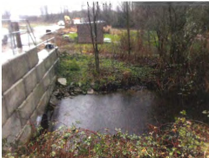
PHOTO 12: LOOKING DUE SOUTH ACROSS THE ENTRANCE OF 17260 RIVER ROAD. THE SOIL PLACEMENT AREA IS LOCATED IN THE TOP LEFT CORNER OF THE PHOTO. THIS CROSSING WAS UPGRADED IN 2019 - THE OLD CROSSING WAS SITUATED TO THE RIGHT OF THIS PHOTO.
