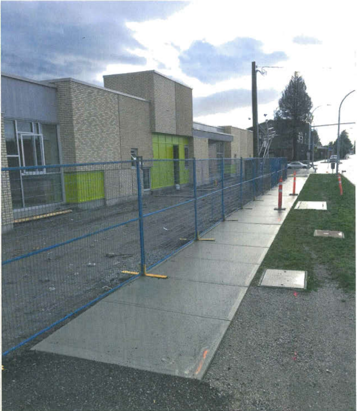
Photo of Building Under Construction
