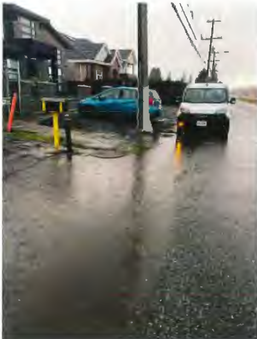
January 24, 2020 - Localized ponding
