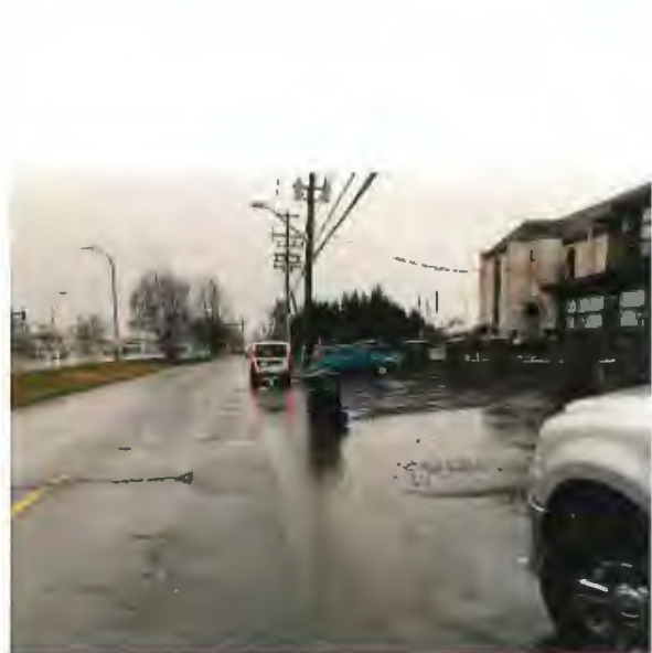
January 24, 2020 – Localized ponding
