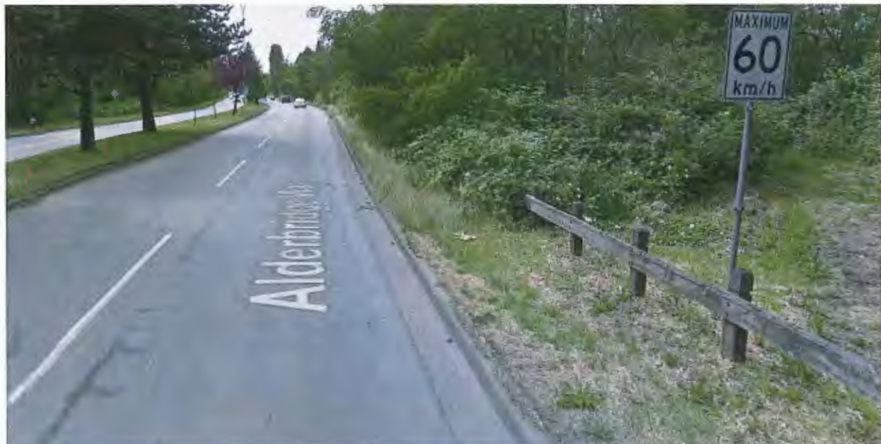
Before: North side (westbound) Alderbridge Way west of Shell Road
