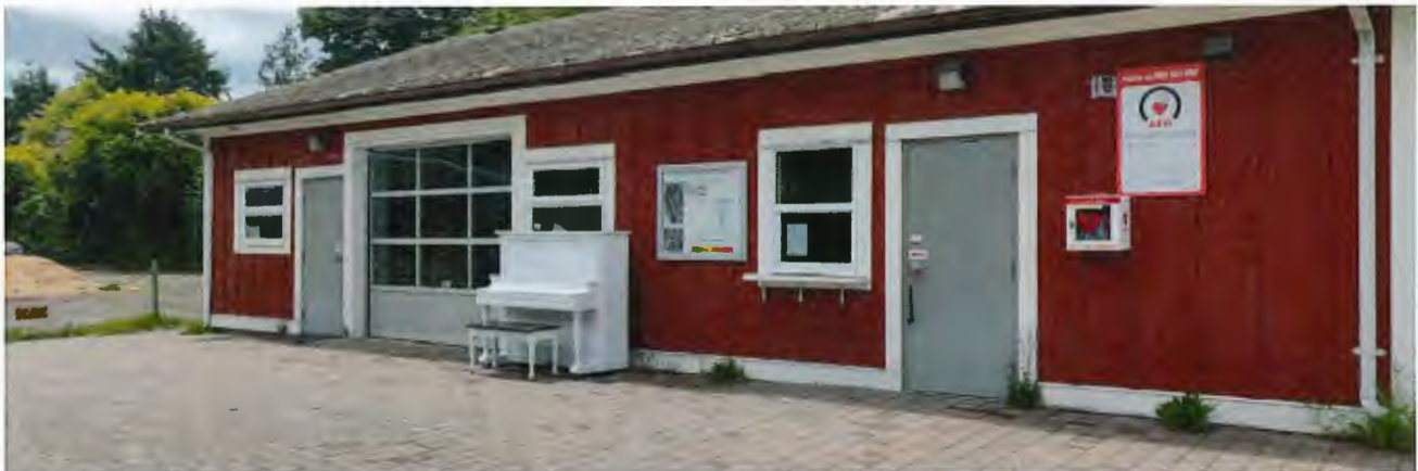
Figure 3. Terra Nova Barn doors provide access to adjacent courtyard
