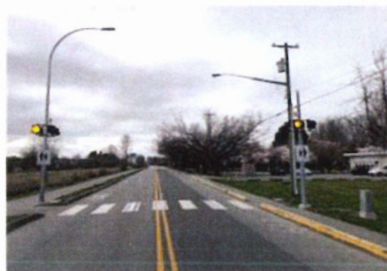
Figure 1: Special Crosswalk on Shell Road at Kidd Elementary School
