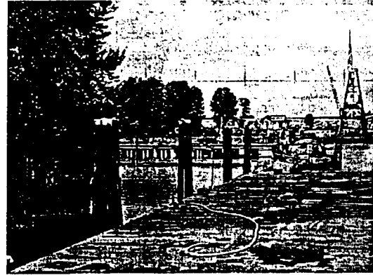
Pier along Queensborough Perimeter Greenway in place at Port Royal
