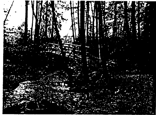
Bridge over Byrne Creek along Byrne Creek Ravine Trails
