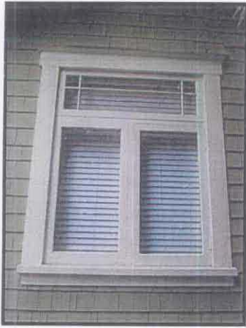
Windows: Wood frame
