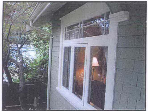
Windows: South east side
