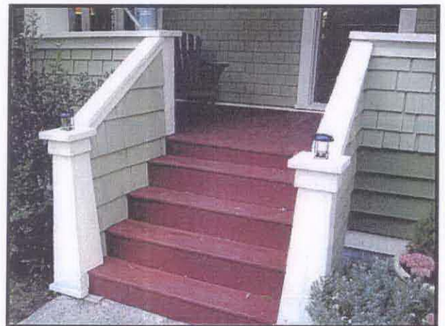
Architectural: Porch, steps
