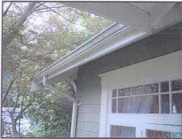
Roofing: gutters & fascia
