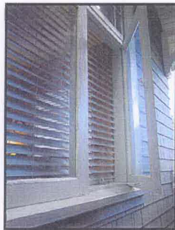
Windows: Wood frame
