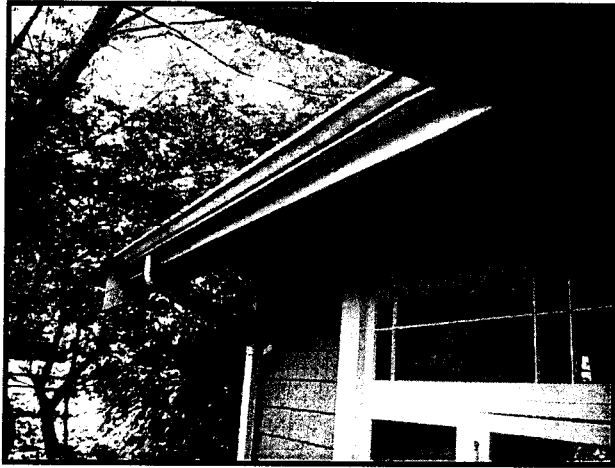
Roofing: gutters & fascia
