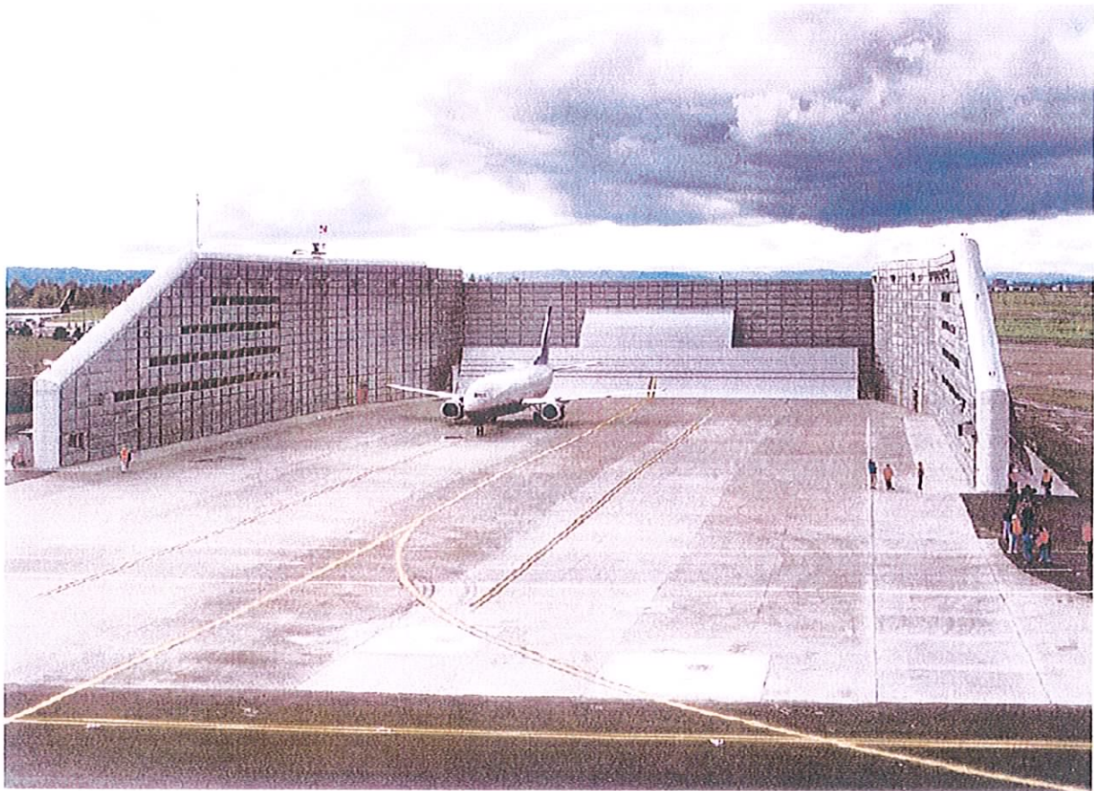
FIGURE 2 Portland International Airport Ground Run-up Enclosure (photograph courtesy of Blast Deflectors, Inc.)
