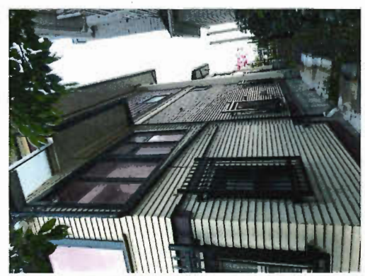
② EXISTING NORTHWEST CORNER
