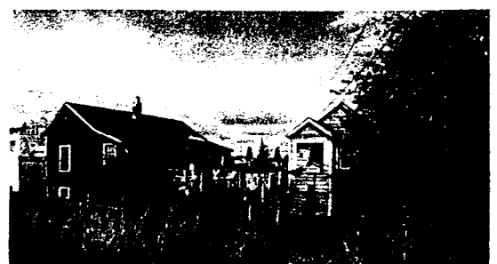
Stilt Pile Housing
