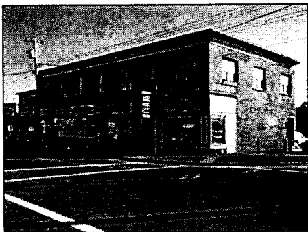
Hepworth Block (c. 1913) at 3580 Moncton Street
