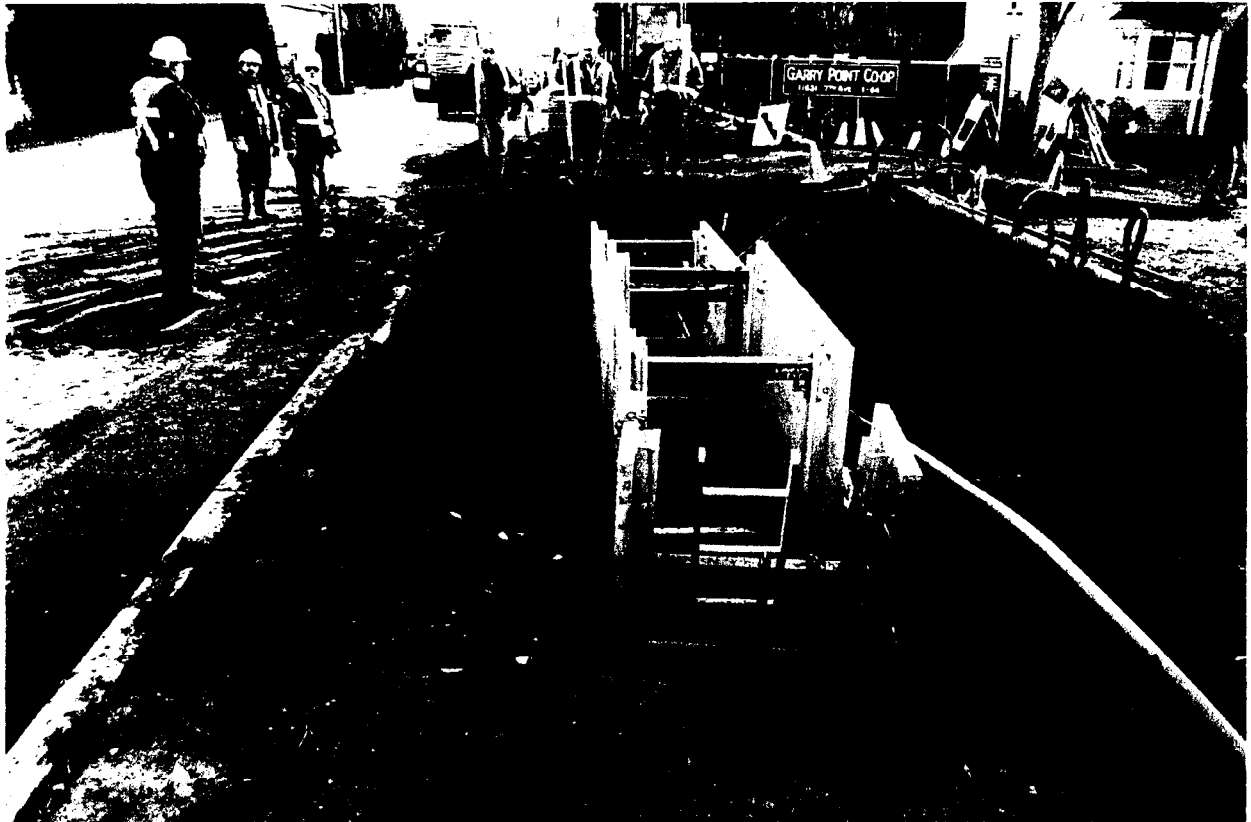
Conventional open cut sewer point repair.
