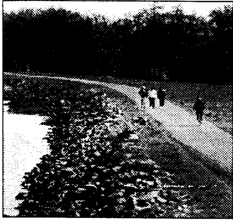
Richmond's dyke system provides floodproofing protection
